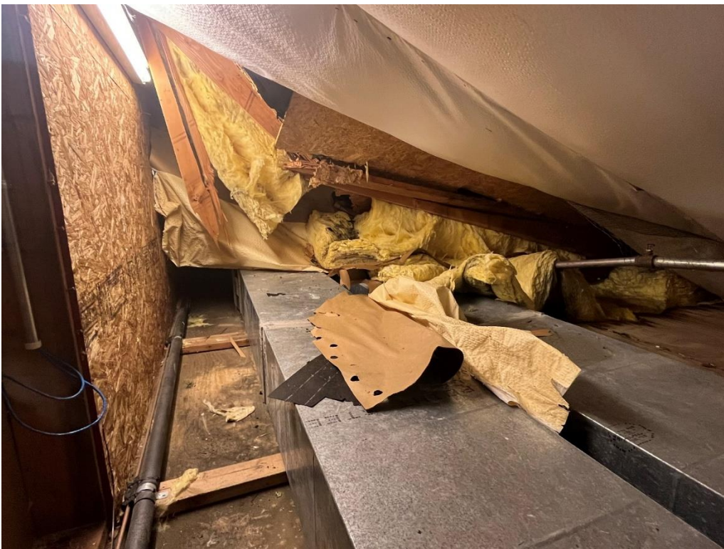
Image 3: Roof of Interstitial Space Looking East
