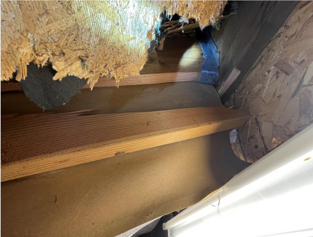
Image 2: Interstitial Space Roof Joist at High Point
