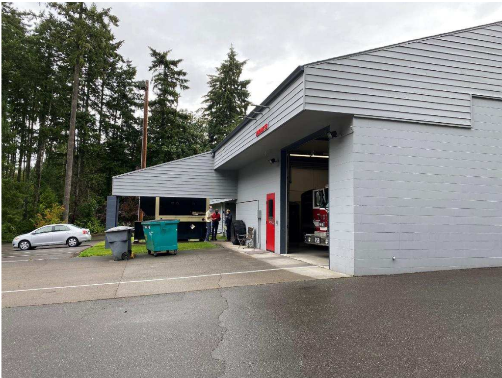
Figure 3.1-2. Fire Station 58 Exterior, Rear of Apparatus Bay.
