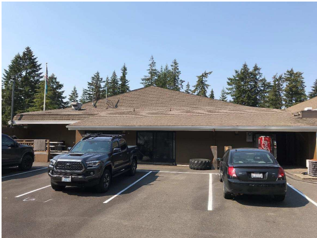
Figure 3.2-2. Fire Station 51, Exterior looking East.
