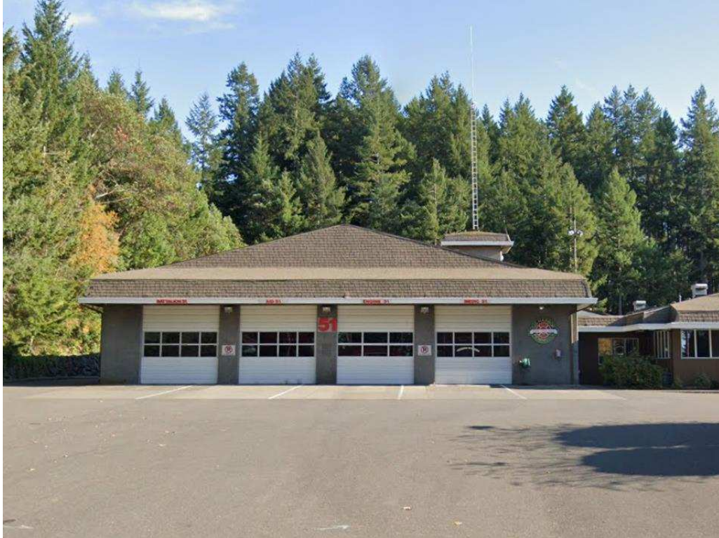
Figure 3.2-1. Fire Station 51, Apparatus Bay Exterior looking West.
