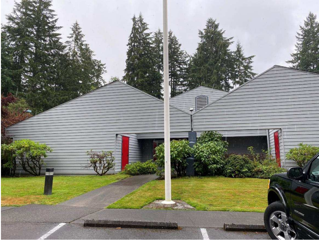
Figure 3.1-1. Fire Station 58 Exterior, Public Entrance.
