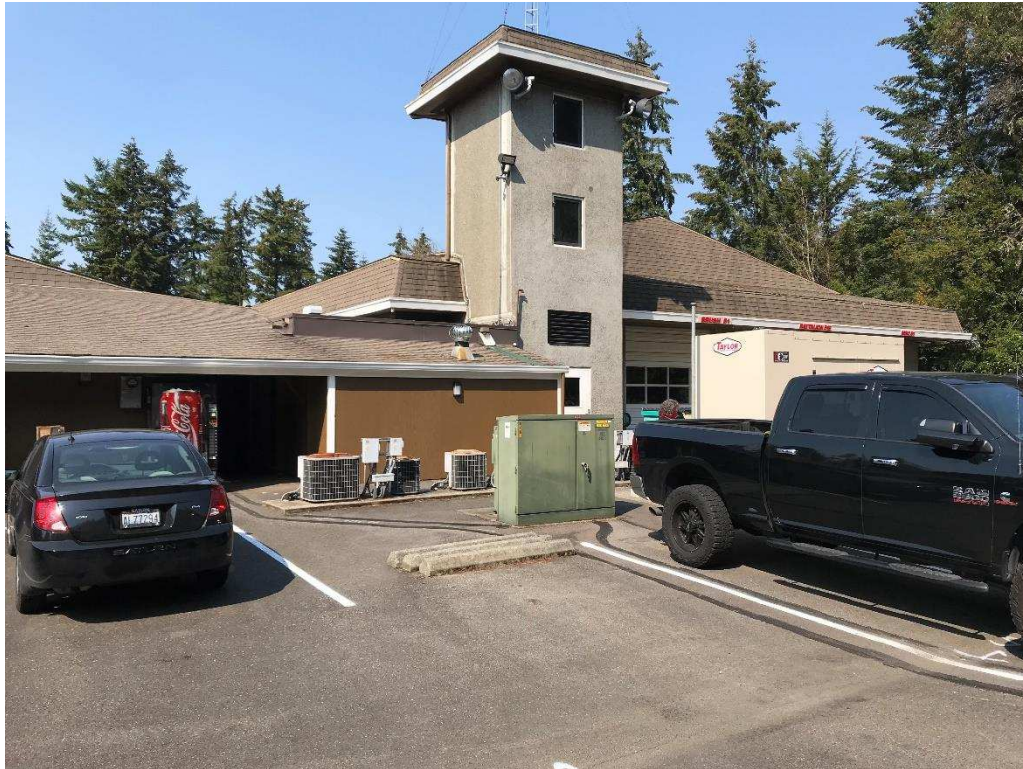
Figure 3.2-3. Fire Station 51, Hose Tower looking Southeast.
